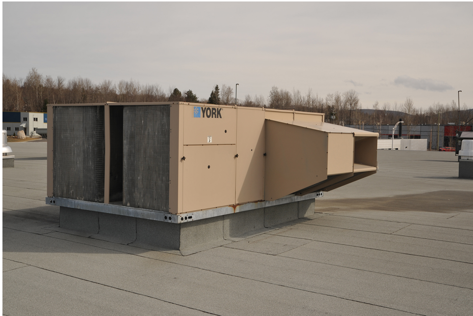
Figure 5. Typical RTU.
