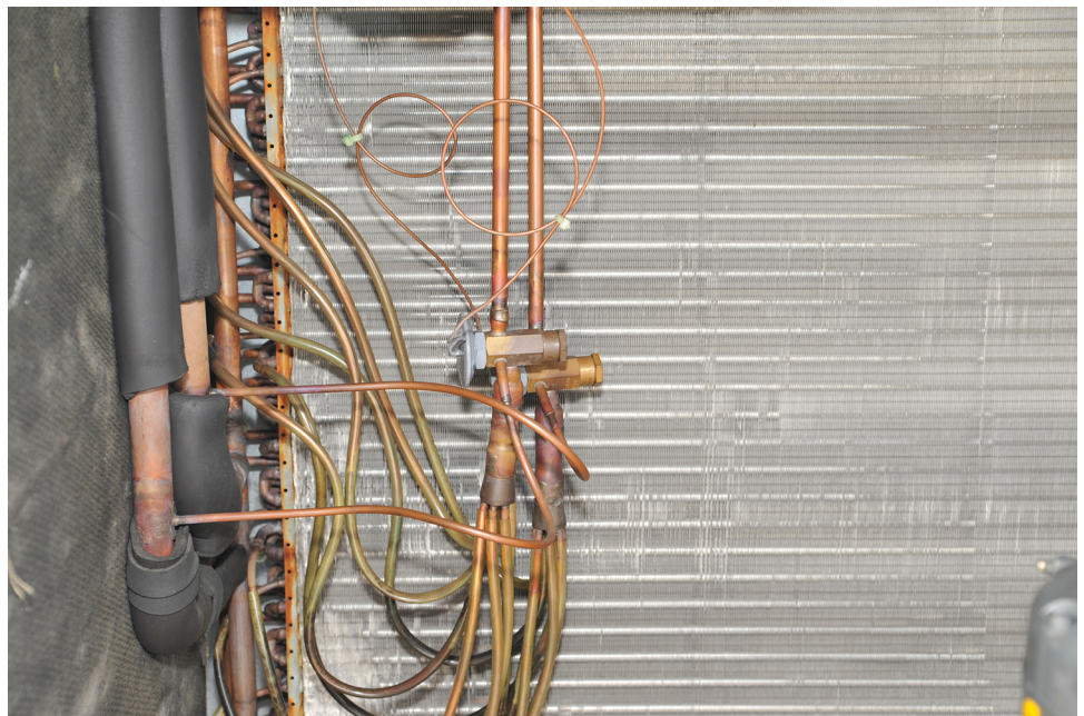
Figure 8. Cooling coil.
