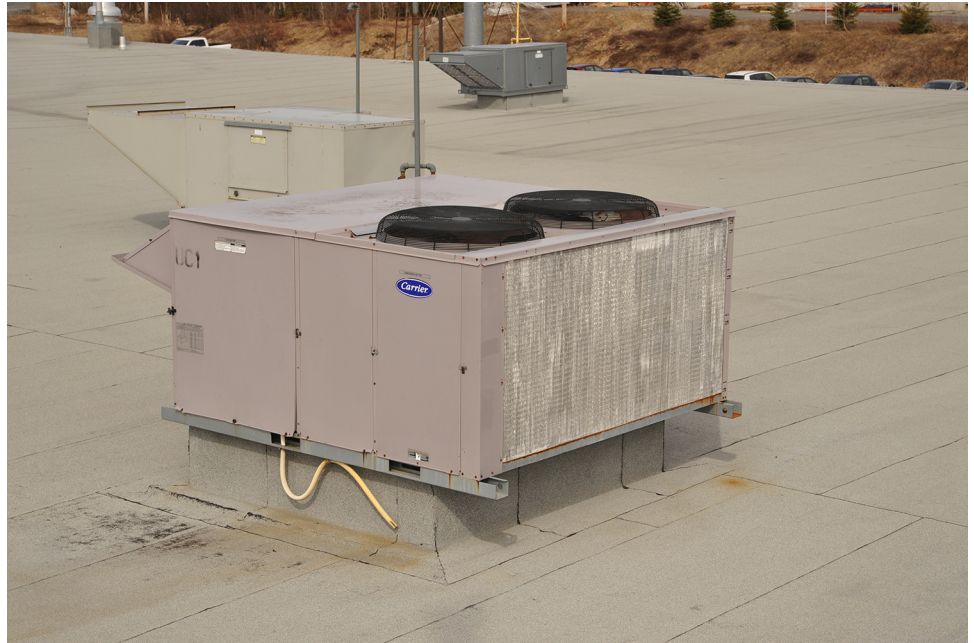
Figure 4. Typical RTU.
